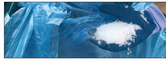
Above: Dry ice pellets used to blast away lead-based paint on the armory stairs. Below, a worker is seen through an oberservation window at the armory, using the dry ice technique to clean the concrete steps.
