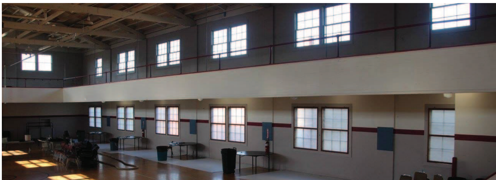
Despite reports from Eugene that note worry over armory lead levels, the city says all precautions are being taken. Pictured: Vintage Window Restoration completing the armory's window project. Photos courtesy of Facebook.
