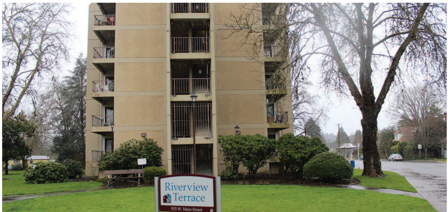
An ongoing investigation is attempting to locate a suspect in a possible arson case after a fire broke out at Riverview Terrace.
