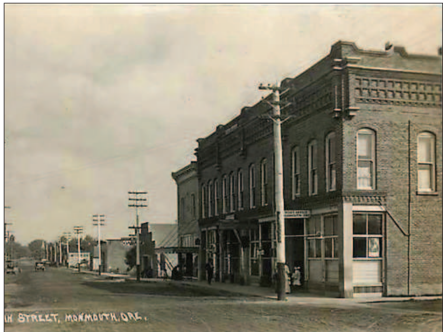
The main street of Monmouth as it appeared in 1915. This location is still readily recognizable today.
