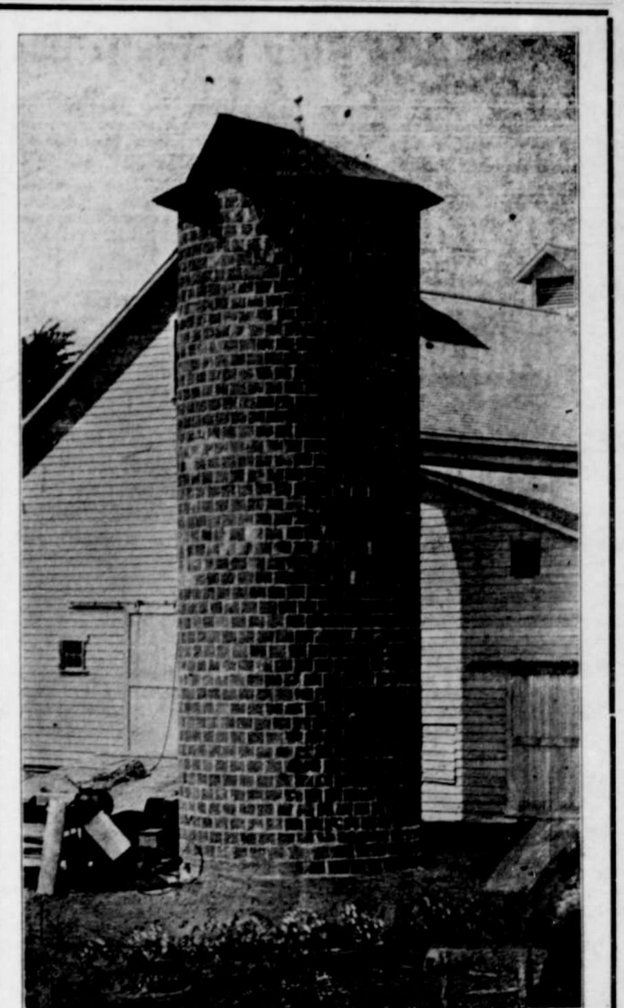
The above is a picture of the hollow tile type of silo such as have been erected on the farms of N. W. White and J. A. Powell on Coast Fork, and for which S. L. Godard is agent. This picture was taken on the farm of Harold Stephens, at Amity.
