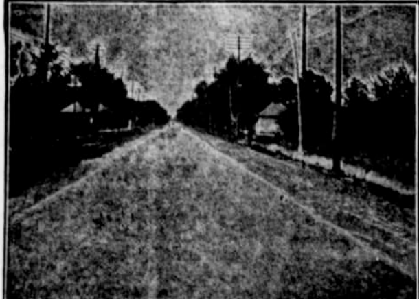
This is the way they will look after being paved with concrete
