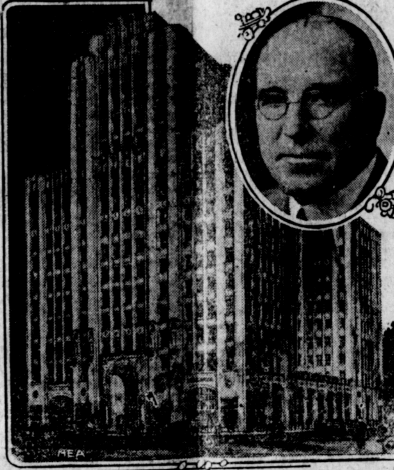
This 14-story temple is being built at Detroit by the Order of Maccabees. Governor Alex J. Groesbeck of Michigan and Senator Royal S. Copeland spoke at the laying of the cornerstone ceremonies for which were in charge of Supreme Commander A. W. Frye (inset).
