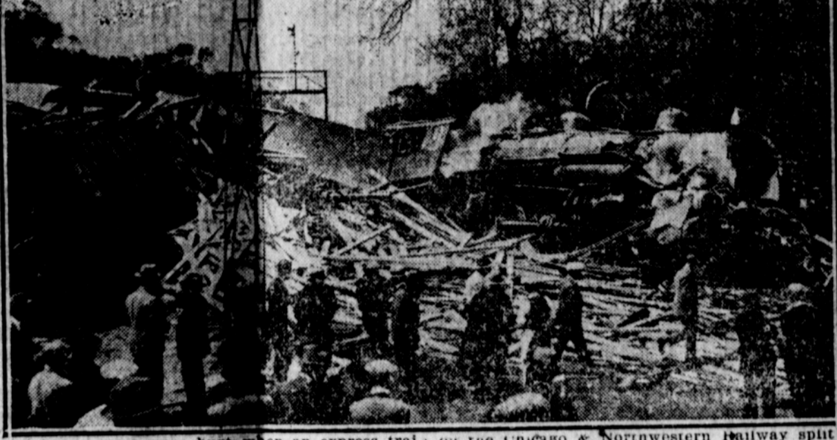
Twelve passengers were hurt when an express train on the Chicago & Northwestern railway split a switch at Wilmette, Ill., near Chicago, and crashed into a freight train on a siding.
