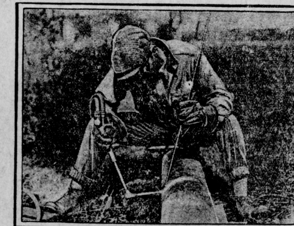
Steel melts and fuses into a solid permanent joint under the intense heat as the welder works.
