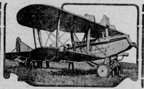
Mechanics at Curtiss field, L. I., tuning up the new "nighthawk" aeronarine plane, especially designed by P. G. Zimmerman for 24-hour flights in he coast-to-coast air mail service in which it will soon make its bow. To nake emergency landing safe it has a low speed of only 44 miles per hour and t is equipped with two powerful searchlights, one on either wing, as shown in photograph. It also has small "riding" lights to prevent collisions and elecrically illuminated instruments.
