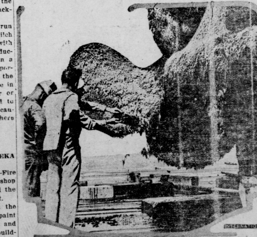
If you think the boys in the navy have an easy life, take a look at this propeller of the U. S. S. Paul Hamilton, in dry dock at San Diego, Cal. It is covered with barnacles and other sea growth and the lads inspecting it will have to help scrape it clean.
