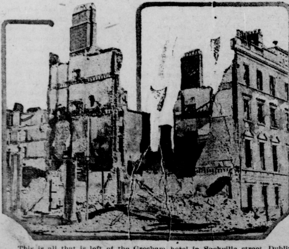
This is all that is left of the Gresham hotel in Sackville street, Dublin, after it had been shelled by the Free State troops to drive out the irregulars, who had their headquarters there.
