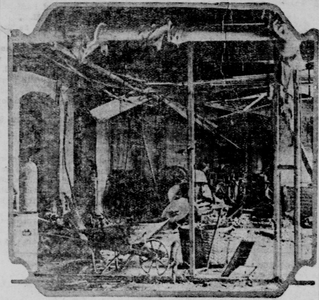
A view of the interior of the Jefferson laboratory at Harvard university that was totally demolished by an explosion which is said to have originated in a gas or oil tank, two men were killed and many were seriously injured.
