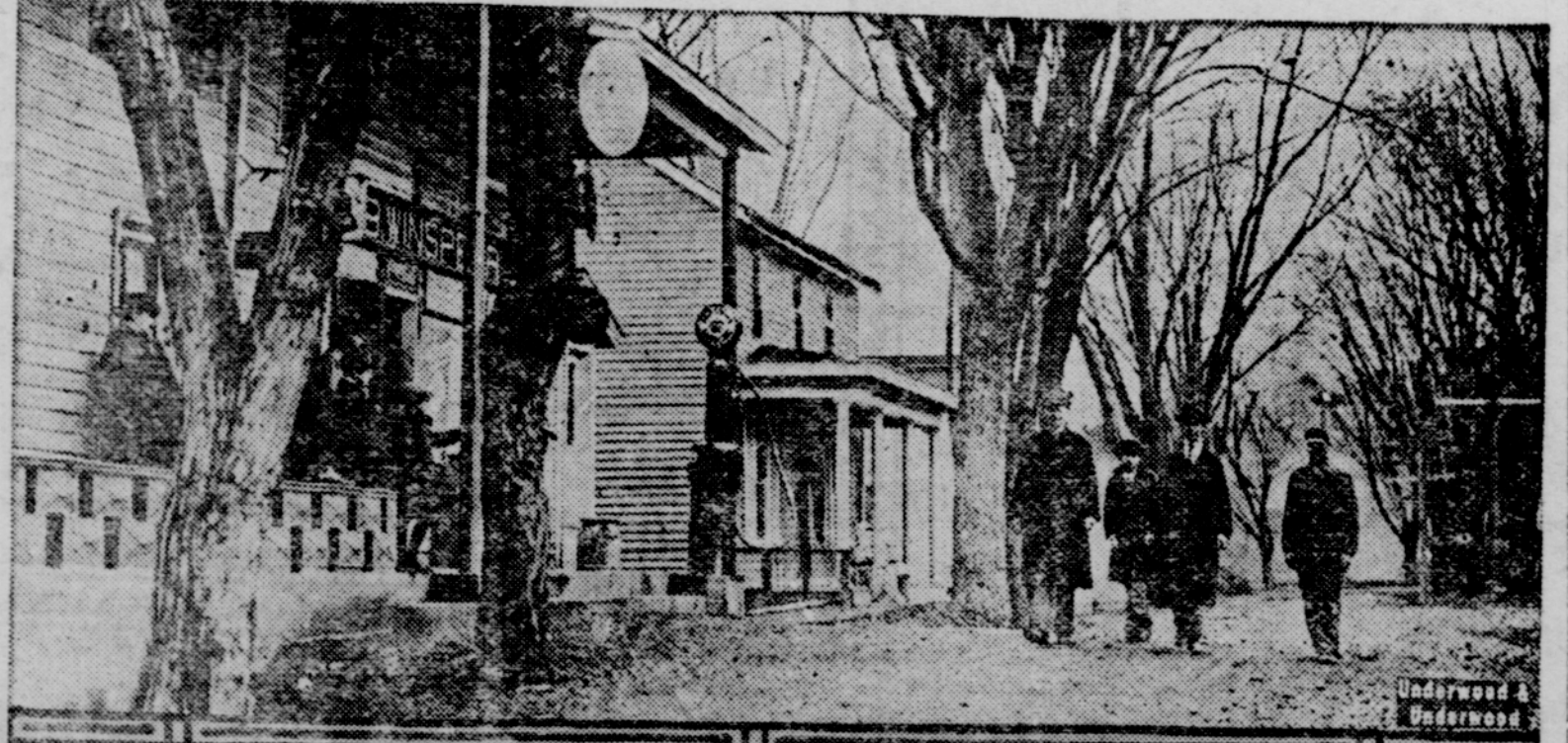
The celebration on April 27 of the centenary of General Grant's birth centers public attention on the town of Point Pleasant, O., where the soldier and President was born. This photograph of the main street of that town shows, at the left, the cement porch from which President Harding will address an audience assembled from all parts of the nation. His speech will be transmitted everywhere by radio.
