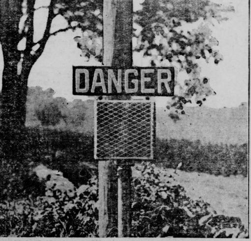
outside the city limits of Boston this glowing radiator casts a reflection as a danger warning to speeding autoists. A hundred yards away there is a sharp "S" in the road, and many collisions entailing serious injuries and loss of lives occurred before the "glow worm" was erected.
