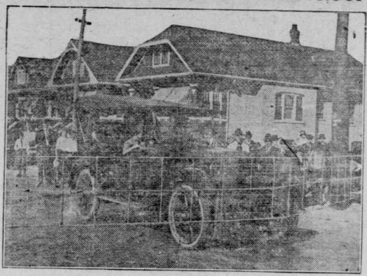
Officials of the Chicago elevated railway lines have tested a new satety gate for railroad crossings which is said to be "fool-proof" against the careless automobile driver who now and then drives through the old-fashioned wooden gate and wakes up with a harp. The new gate will not allow an automobile locate the missing cars, when the to pass. If a car runs into it the gate gives several feet and then bounces the car back like a rubber ball.
