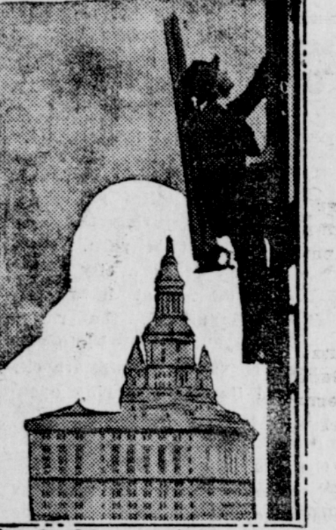
CLIMBING N.Y. CITY'S TALLEST CHIMNEY TO OBTAIN UNUSUAL SHOTS OF MUNICIPAL BUILDING
