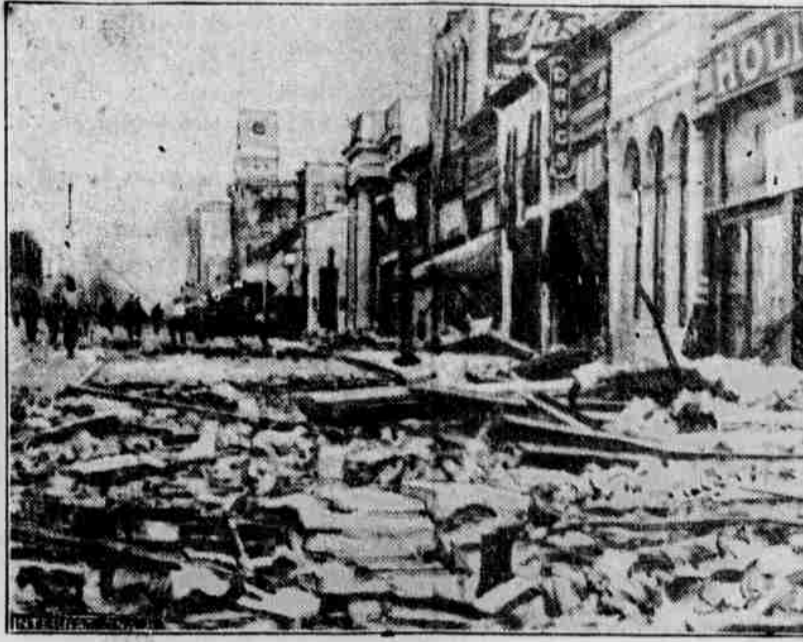
This picture of the wreckage in State street, Santa Barbara, Cal., was made immediately after the first earthquake shocks that shattered that beautiful city. It was transmitted over the wires of the American Telegraph and Telephone company.
