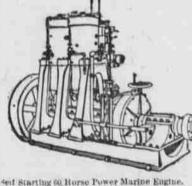
Using gasoline or cheap distillate oil. Engines connected direct with propeller shaft, and no noisy, easily broken bevel gears used in reverse motion. New spark device; no internal sprins electrodes to burn out.
