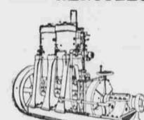
Using gasoline or cheap distillate oil nnected direct with propeller shaft, and no notsy, easily broken bevel gears used in reverse motion.
