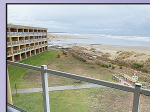
88416 1ST AVE B UNIT Florence's only oceanfront condo complex: Driftwood Shores. This popular "B Unit" on the 3rd floor. It features 2 BR/2 BA and 780 SF w/ balconies overlooking the beach. Recent interior upgrades include granite counters, custom tile showers, flooring and furnishings. $188,500 #11943 MLS#20616254
