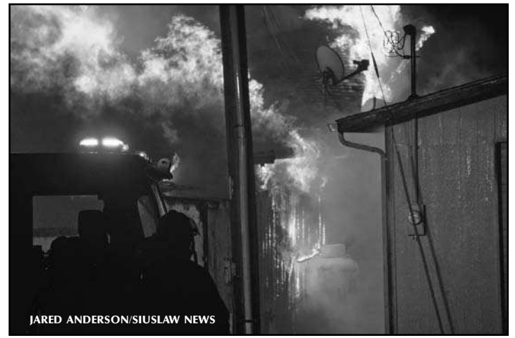
The March 1 blaze at the former La Bu La Restaurant left only a shell of the building which has housed multiple businesses over time.
