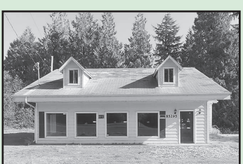
85295 Hwy 101 – Highway frontage and exposure! Nearly 1,000 sqft of retail space, with large store front windows, 8'x10' truck door, and second buildable lot for parking or expansion. This building is fully ADA-accessible including the restrooms. $150,000. #2784-17074277
