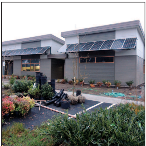
The new Public Works Facility provides more efficient work space.
