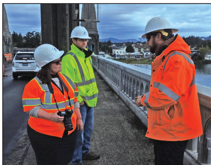
From left, ODOT Public Information Officer Angela Beers Seydel, Project Coordinator Shane Prohaska and Senior Inspector Nathan Neal tour the Siuslaw River Bridge Cathodic Protection Project last week. “It’s what I love about my job — days like this,” Beers Seydel said.
