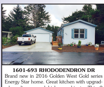
1601-693 RHODODENDRON DR Brand new in 2016 Golden West Gold series Energy Star home. Great kitchen with upgraded appliances and hickory cabinets. This 2 bedroom, 1 bath home has a ductless heat pump/ air conditioner with additional forced air heat. The bath is senior friendly, with a step-in shower and hi-rise toilet. 2 car garage and a low-maintenance lot that's nicely treed and has sunny exposure. $157,900 #11390 MLS#16347585
