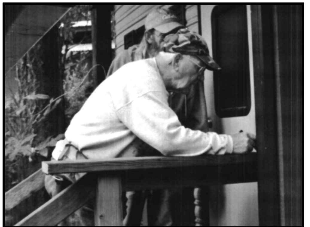
Ray Dunning and Sam Lewis building a wheelchair ramp.
