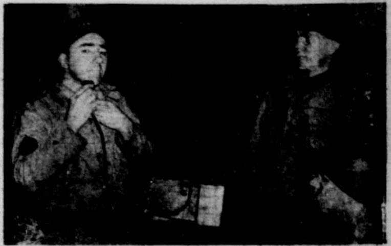
Trailblazer Photo TEC4 GEORGE NIKOLAI demonstrates his bivouac-model electric shaver to Tec4 Victor Nygren and Pvt. William Skou (right). It operates off discarded dry-cell batteries through a special socket arrangement which he devised.
