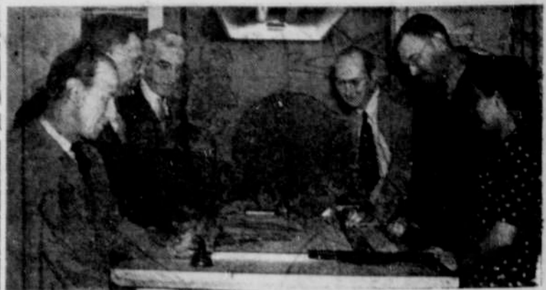
GATHERED ROUND A drafting table at the Post Engineer office are a few of Camp Adair's "original" employees. As members of the U. S. Area Engineer's staff, they moved to Adair from Albany on Mar. 8, 1942, setting up shop in what is now Post Headquarters, the only completed building at that time. The group includes (l. to r.): Frank Haberle, draftsman; Chet Lynds, plumbing foreman; Royal Berry, property section; Frank Koehler, engineer; Warren Clarke, electrical foreman; Betty Gunther, property section.
