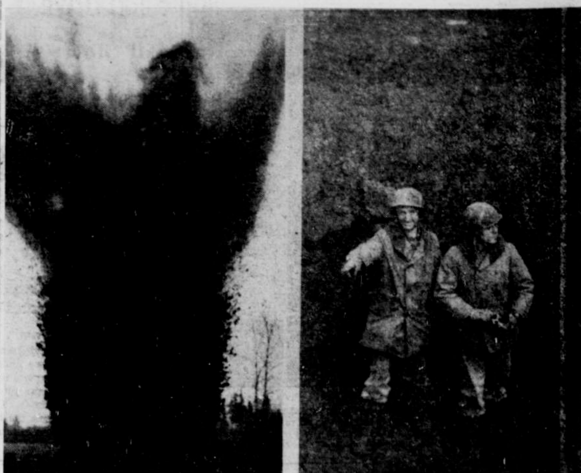
TONS OF ROCK and debris (left) form a fountain against the sky as 200 pounds of explosive blast a road block for the 316th Engrs. in a recent demolition problem. The earth flew more than 300 feet into the air. At right, Sgts. Edmund Wasielewski and John H. Gonzales examine the crater left by the explosion. It was 30 feet in diameter and over 12 feet deep.
