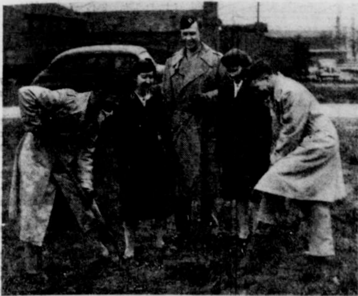
MR. WILLIAM E. GRAINGER, JR., field director at Camp Adair for the American Red Cross, and Capt. Gilbert A. Waite, Post director of personnel, share the honors in digging out the first shovelful of earth on the site of the future Red Cross administrative headquarters building on Theater Avenue. Looking on are (l-r) Miss Ada Keyes, Red Cross administrative assistant field director, Capt. Howard L. Preston, Post engineering operations officer, and Mrs. Davida Marsh, Red Cross claims staff aid.
