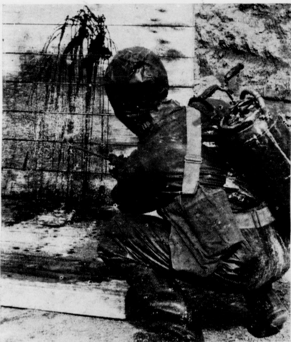
A MEMBER OF a Chemical Warfare decontamination squad works on a simulated wall area that has been contaminated by a vesicant gas. Using the standard three-gallon spray apparatus which contains a slurry of chloride of lime and water, the man is carefully spraying the entire contaminated area. This same treatment is used on any contaminated wooden surface except floors.—Signal Corps photo.
