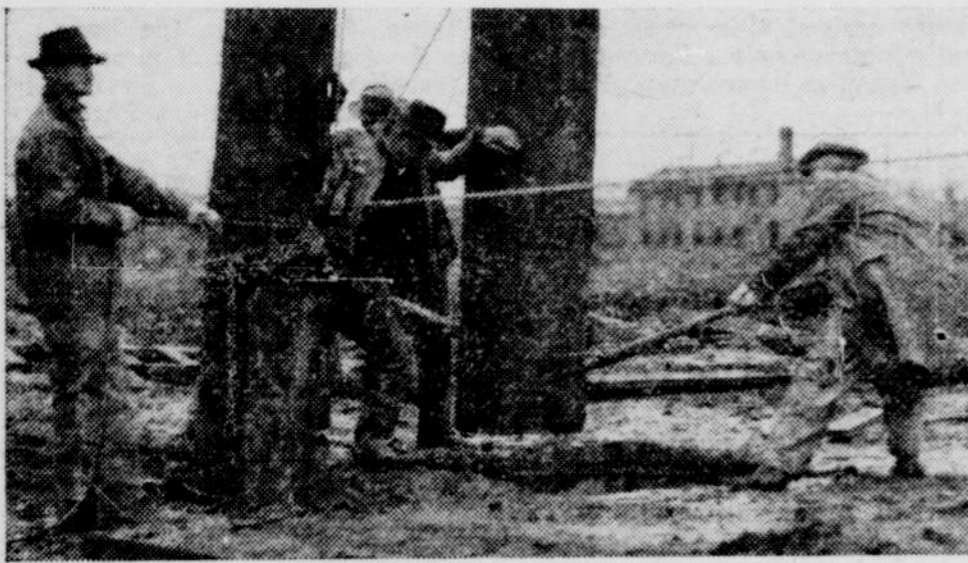
The pole is shown here hoisted and "dead over dead center." The critical stage passed, workmen of Post Engineers are ready to drop it into its concrete filled bed. —Public Relations Photo.
