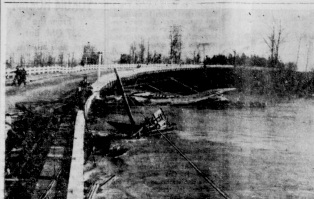
Once upon a time it rained and rained in Oregon. Proof is hereby presented in a photo that recently arrived by ex team. It shows the Mellow Moon dance hall and roller rink resting uncomfortably under the West Salem bridge. The bridge has since been repaired. The Mellow Moon, alas, is no more.
