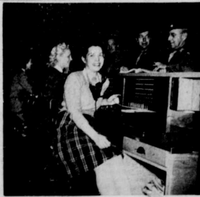
Behind the switchboard at the new Camp Adair Service Men's Telephone center. The smiling operator in the foreground is Meiva Golden. Just behind her is Bernita Edmondson and then Mary Dickhouse. Story on page six.
