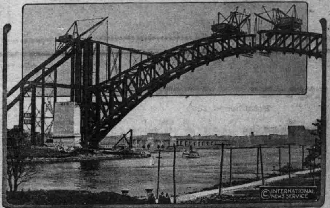
When the last girder of the 19,000-ton bridge over Hell Gate, New York city, was put into place recently, the largest, heaviest and most expensive structure of its kind in the world was nearly completed. The bridge, built for the New York Connecting railroad, is 1,017 feet long and its cost is $12,000,000.
