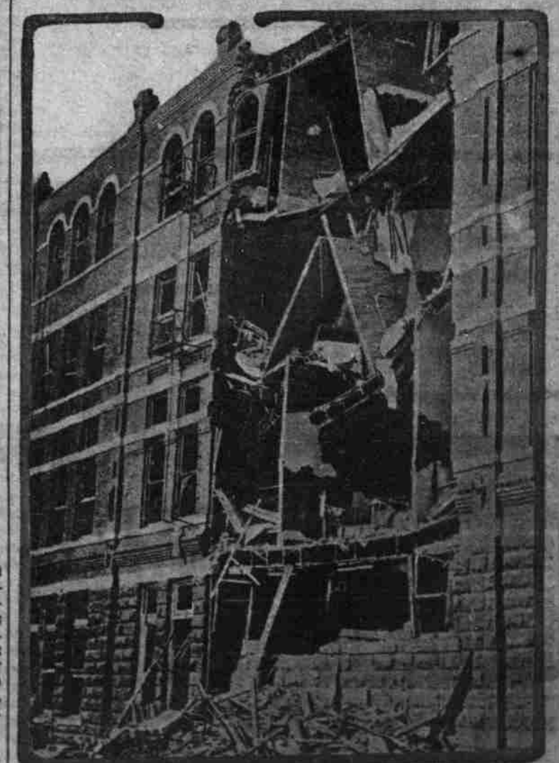
Many persons were killed or injured and great damage done to property in Ardmore, Okla., by the explosion of a tank car of gasoline and the resulting explosion of a quantity of dynamite in the railroad yards. This photograph of the east wall of the Whittington hotel shows how numerous buildings were shattered.
