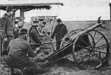
This novel instrument is used by the French to cut barbed wire entanglements in front of the German trenches. The gun throws the hook into the midst of the wires and a cable that is attached to it is then recied in, bring-
