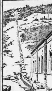
Mountain Stream Conducted Through 30-Inch Pipe to Hydro-Electric Plant.
