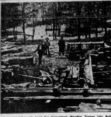
Portable Sawmill Used for Converting Woodlot Timber Into Switch Ties, Which Are Extra Long-The By-Product of Such Ties in the Form of Stabs and Edgings, With Some Boards, Can Be Utilized for Lumber. Near Dubuque, Iowa.
