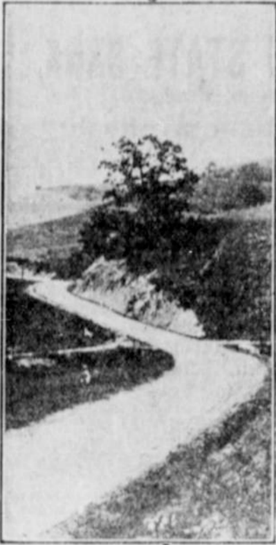
THIS ROAD WAS LOCATED AND CONSTRUCTED BY A COMPETENT HIGHWAY ENGINEER.
