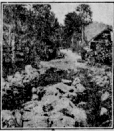
THIS ROAD WAS REPAIRED UNDER THE STATUTE LABOR SYSTEM.
