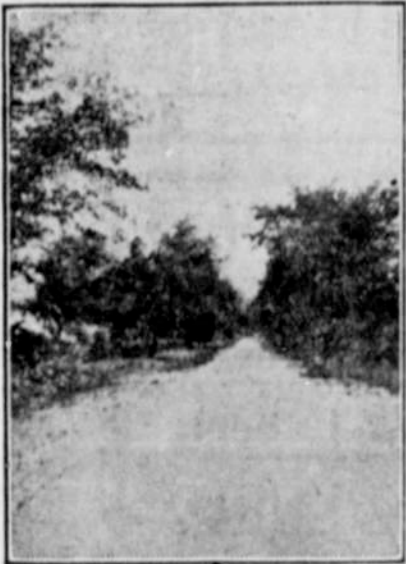
A STATE AID ROAD IN NEW JERSEY.
