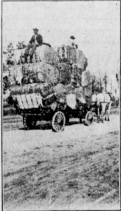
WELL BUILT MACADAM ROAD—MAXIMUM LOAD FOR TWO HORSE TEAM, TWELVE BALES OF COTTON, 5,000 POUNDS.
