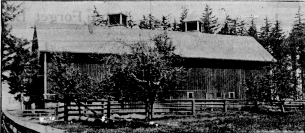
Typical Livestock Barn of the Rockwood Region
