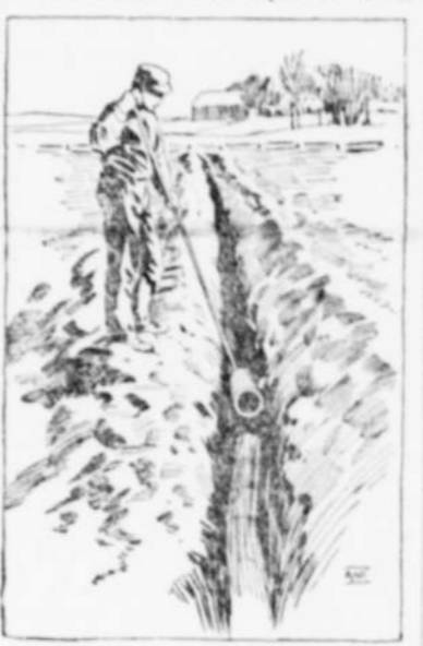
FIG. 2—POOR WAY TO LAY TILE.
