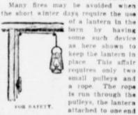
and then pulled up to a convenient height, the loose end of the rope being fastened to a cleat on the wall. If this device is arranged in about the center of the barn much better light will be given than if the lantern were carried around from place to place. Cor. of Farm and Home.
