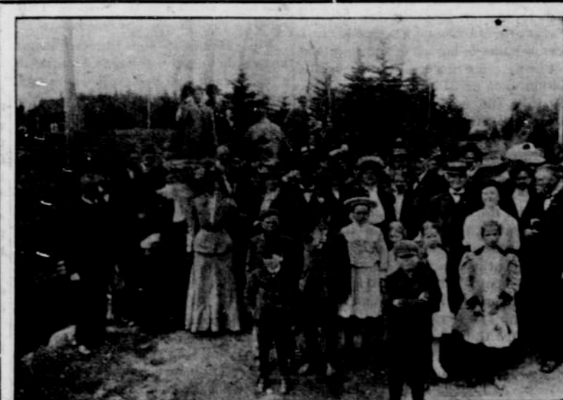
Taken at Official Opening of Fairview Branch O. W. P. Electric Railroad, June 29
