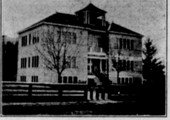
GRESHAM PUBLIC AND HIGH SCHOOL BUILDING
