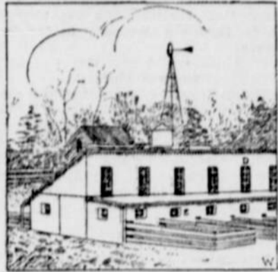
FIG. 1.—VIEW OF PART OF HOG HOUSE
