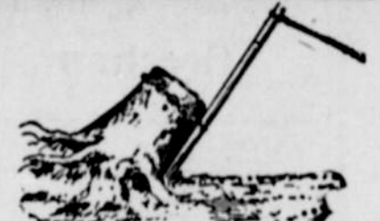
FOR PULLING THE STUMPS.
