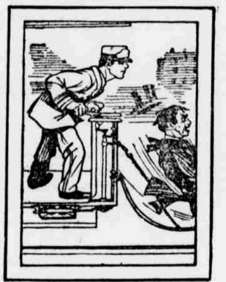
FENDER DROPS CLOSE TO THE GROUND.
